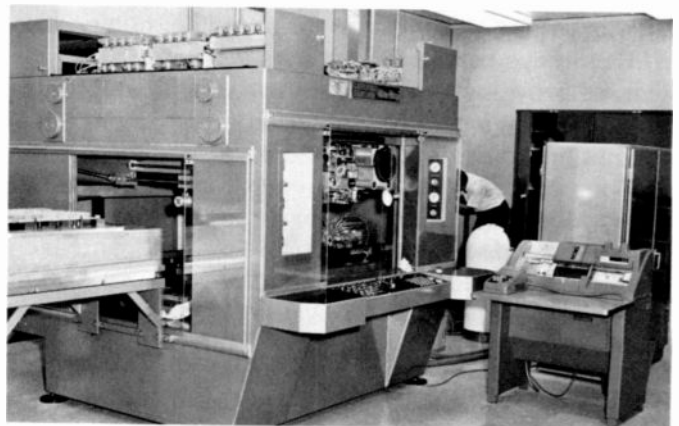
Fig. 1. Gardner-Denver automatic wire-wrap machine
