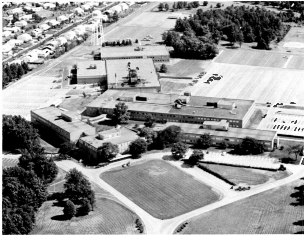
RCA Service Company Headquarters, Cherry Hill, New Jersey.
