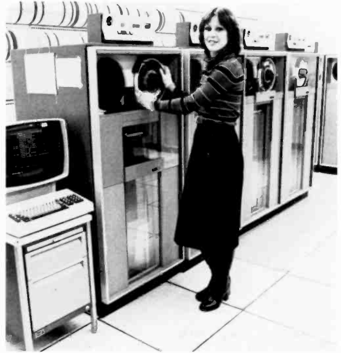
Fig. 2. Shown are the IBM 2177 display station and 3400 tape drives. The tape librarian is demonstrating the mounting of a tape for processing by the system.
