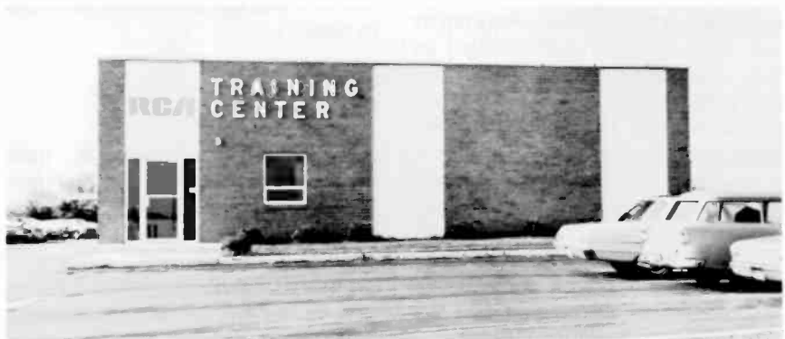
Fig. 3. There are approximately 165 RCA Service Company Consumer Service branches located in major cities throughout the country.
