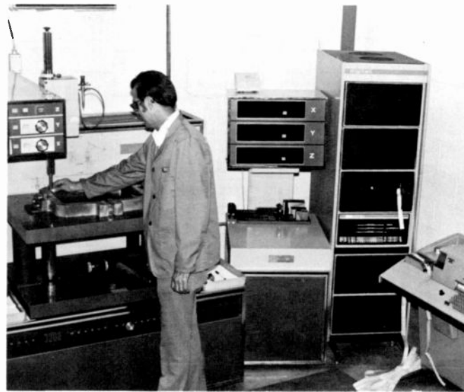
Cordax gaging system—measuring the periphery of a shell.
