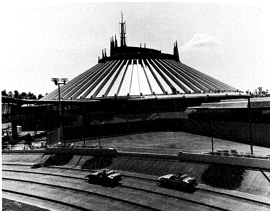
Space Mountain dominates the Tomorrowland area at Walt Disney World. The ribbed beams that comprise the roof stand out in bold relief to create an attention-getting pattern. (Copyright Walt Disney Productions.)
