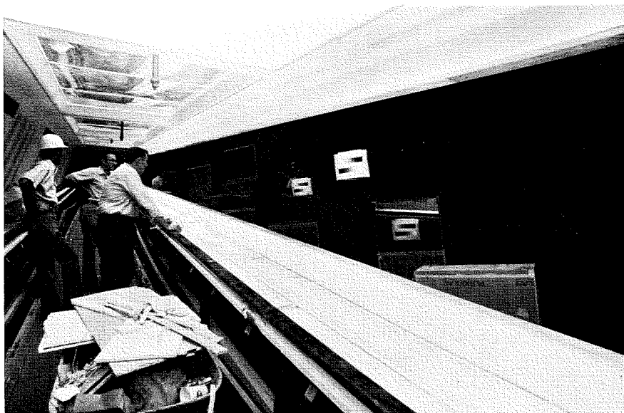
TV area under construction. Jim Cravens, Service Company; Paul Crookshanks, CE, and Greg Bell, Disney (right to left) during the first tests of tv receivers in place.
