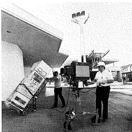
One of the RCA TK-45 cameras and control rack are shown in front of Space Mountain, on their way in for installation by Ralph Olweg (1) and Oscar Klampfer (r), Communications Systems Div. (Copyright Walt Disney Productions.)
