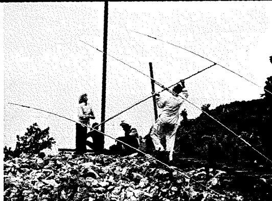
Miles Brown (left) and Joe Duffin (right, coveralls) with two Jamaican crew members erecting a tri-band beam antenna for 14-, 21-, and 28-MHz operation.
