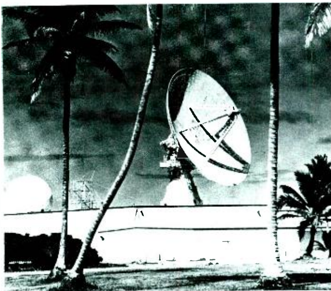
View of the completed TRADEX facility on Roi-Namur Island, Kwajalein Atoll, showing the 84-ft diameter Tracking Radar antenna.
