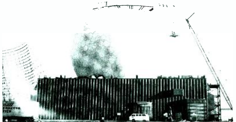
Erecting the 140-ft diameter Tracking Radar radome at the Clear, Alaska BMEWS site.
