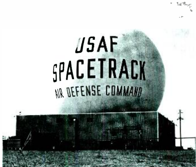
Completed Spacetrack Facility at Moorestown, New Jersey, as viewed from the N.J. Turnpike, showing the 140-foot diameter radome surmounting a three-story structure.
