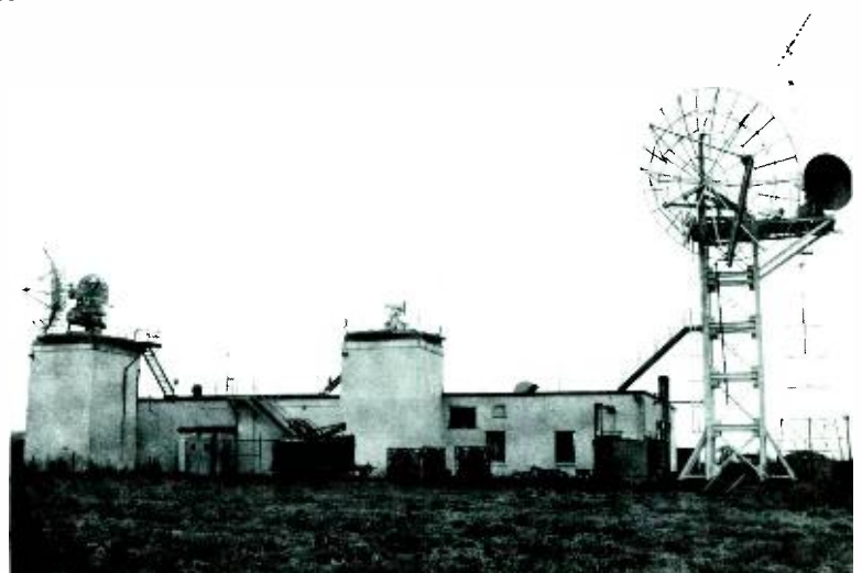
Fig. 3—Antenna laboratory building.
