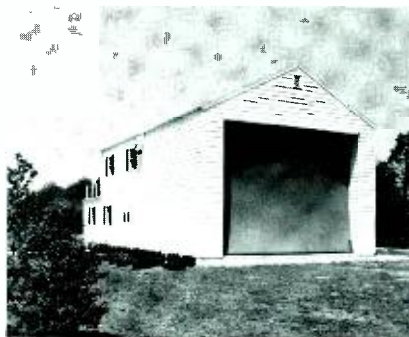
Fig. 1—Antenna development facility at Deptford. The curved radio-transparent wall will be used for "indoor" testing of antennas is at this end of the building.
