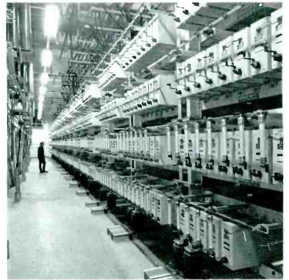
Fig. 8 — Capacitor-bank room.
