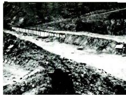
Fig. 7—BOSS test configuration showing containment duct.
