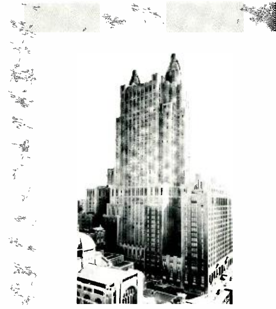
Waldorf-Astoria Hotel, New York City, represents one of the first and most outstanding installations of the RCA Antenna Systems and RCA Victor TV Receivers.
