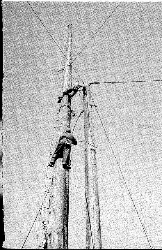
Setting up a rhombic antenna apex pole (Rocky Point).
