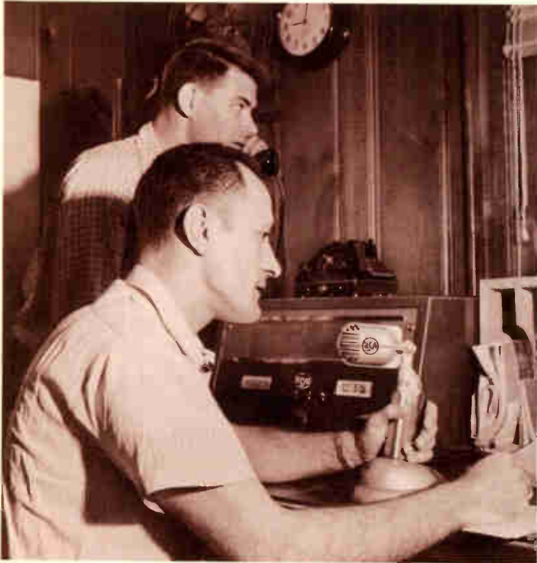
9:01 A.M. WELLPOINT GENERATOR AT WOODMERE IS REPORTED BURNED.
