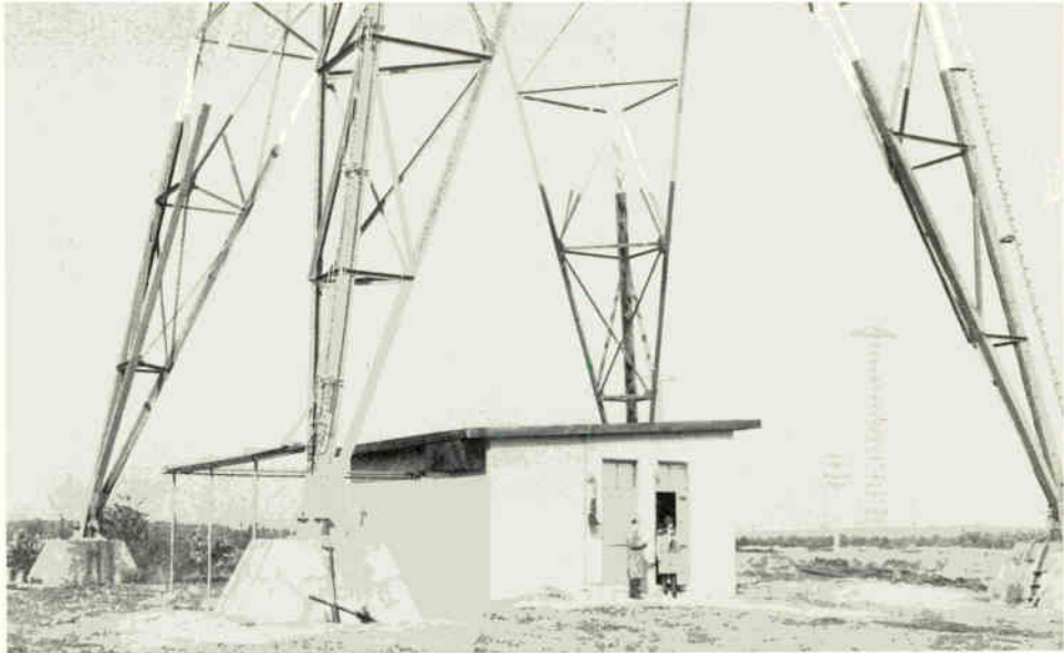
Fig. 1—The Rocky Point microwave equipment is housed in this shelter against a background of overseas transmitting towers.
