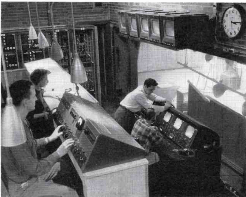
FIG. 5. Television control room overlooks the studio area. Camera, audio and switching controls are located here. Platform at the rear of the control room gives program director and audio operator full view of the studio.
