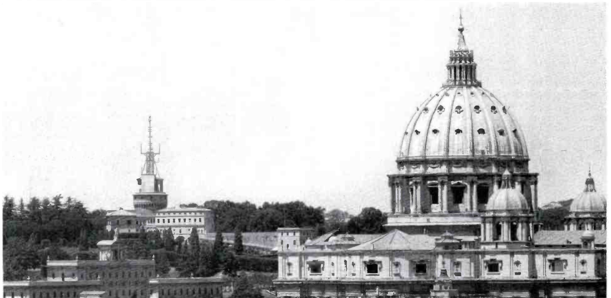
FIG. 3. View of Vatican City, showing St. Peter's at right, and Leonine tower with radio mast and studio to the left.
