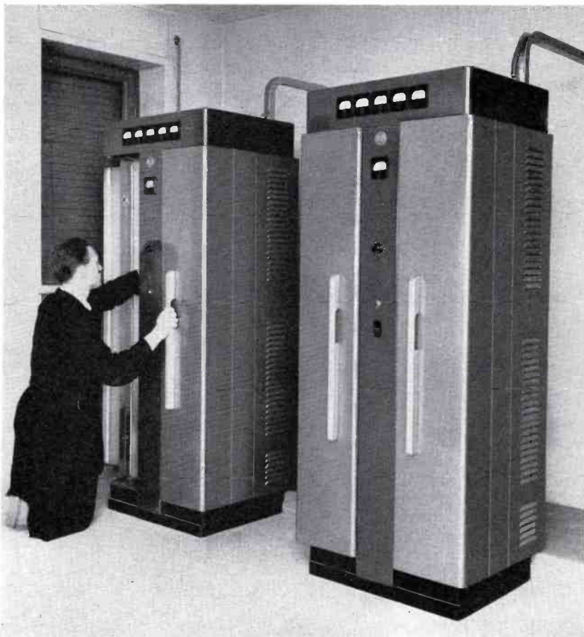
FIG. 28. Two RCA 250-watt FM transmitters are used for local (Italian) broadcasting by the Vatican.
