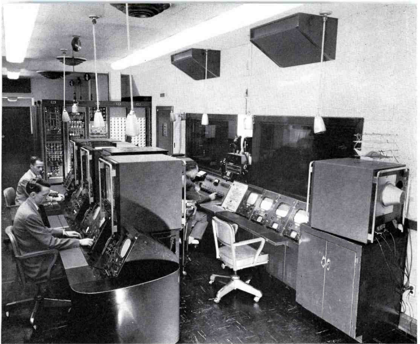
FIG. 15. WBTB's main control room. Master audio and video switching facilities are concentrated in the low console at the right (just in front of the windows which look into the announcers' booths and the studios). Camera control operations are performed at the console, at the left, which contains controls and monitors for all live cameras, film cameras, and Chromascan units. Equipment racks are located at the two ends of the control room. The floor plan of this control room is shown in Fig. 16, on the opposite page.
