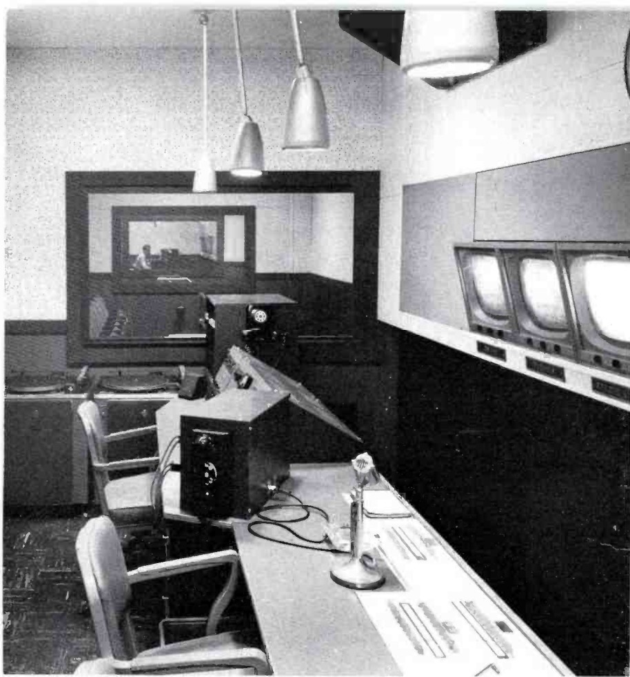
FIG. 22. TV studio control booths and clients' booths are arranged in a line on second floor (see Fig. 9, Pg. 39). Director sits at near position, does his own switching. This view is from TV-1 control room and looks through three double-glazed windows into TV-2 control room 74 feet away.
