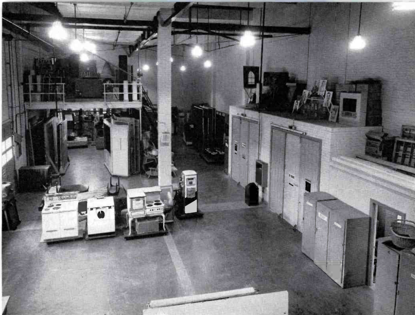
FIG. 10. This large (40-foot by 120-foot) prop construction and storage area is a feature of the WBT-WBTV Building. Large folding doors, at the right, open directly into the two tv studios. Overhead doors, at the left, open onto a loading dock and ramp. This area has the same ceiling height as the studios. Footings, which can be seen in the floor of this area, make it possible to enlarge either or both studios in 20-foot increments by moving non-load bearing studio wall to use part of present prop area.
