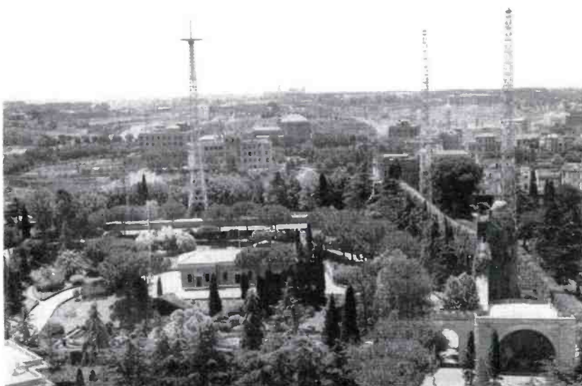
FIG. 24. Vatican transmitter building, showing partial view of antenna system. This building houses eight transmitters.
