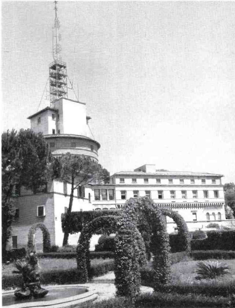
FIG. 11. Antenna system atop studio building for FM broadcasting, mobile link, and STL in that order from top down.
