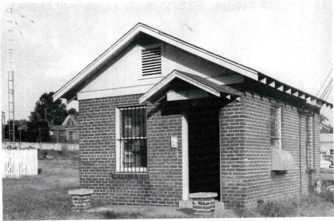
FIG. 8. Transmitter building contains a remotely controlled RCA B7A-1M AM Transmitter.
