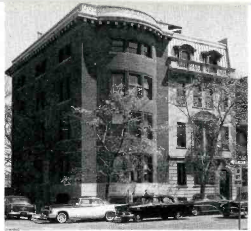
FIG. 14. The Centre is located on the second floor of this building at 25 Granby St.
