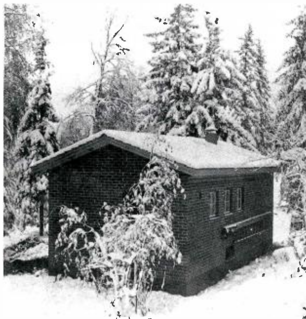
FIG. 5. Koli FM station houses two BTF-3B transmitters—one is a standby.
