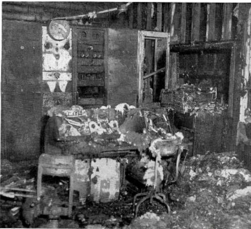
Fire damage in the WCOV-TV studio. One of many scenes of devastation throughout the building. Station back on air in twenty days with new RCA equipment.
