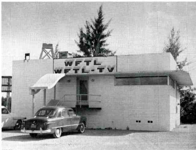
FIG. 8. Exterior view of transmitter building located at 1785 Southeast 15th Street, Fort Lauderdale.
