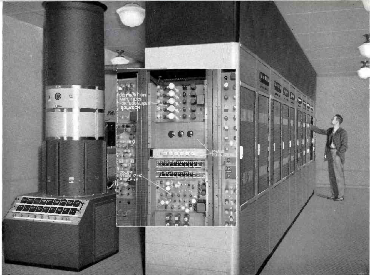
FIG. 1. Conversion to color mainly consists of adding some rack mounted input equipment as shown in the inset of the above photo. This equipment is installed external to the transmitter.
