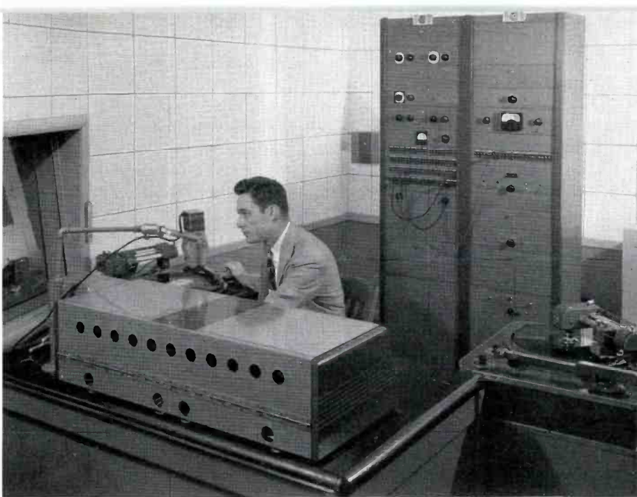
FIG. 2. The Master Control room includes RCA Console, 70 series turntables, recorder attachments and equipment racks. Announcer Jack McKee is at the console controls.
