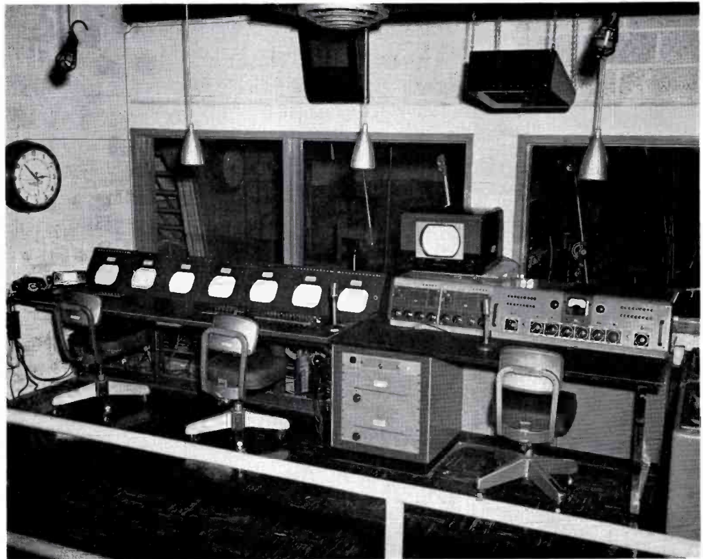
FIG. 11. View of Control Room "A" showing the WOR-TV Program Director's Console at left and the Audio Console at right.
