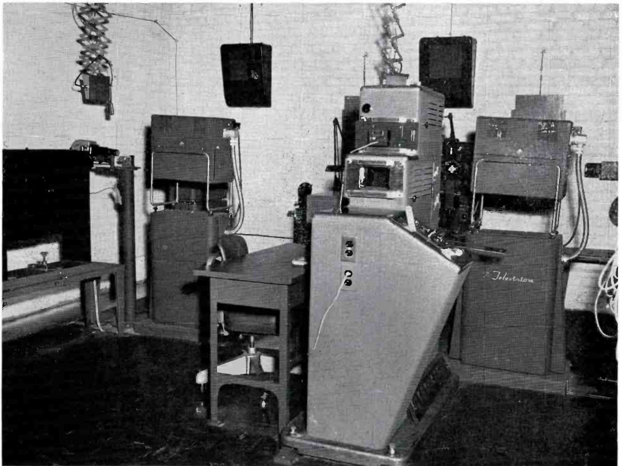
FIG. 26 (below). Another view of Projection Control Room showing location of other equipment. Two RCA TK-20 film cameras with Gray Telop are visible in foreground.
