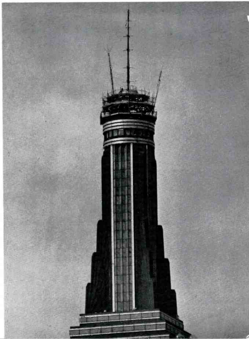
FIG. 1. View of the top portion of Empire State building showing temporary antennas located at each side. Note that photo was taken before old 67-foot TV antenna (center) was taken down. The three platform working levels provided are visible. Photo was taken from the Metropolitan Life Insurance Building with a 40-inch telescopic lens.
