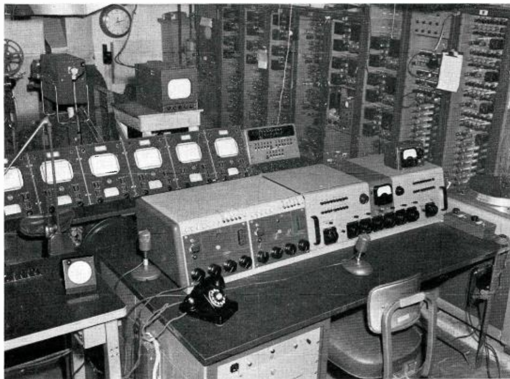
FIG. 42. View of the Program Control Room at the New Amsterdam Theatre. The video console is at a level lower than that of audio console. Sync Generators, Stabilizing Amplifiers and associated equipments are located at the right in fourteen equipment racks.
