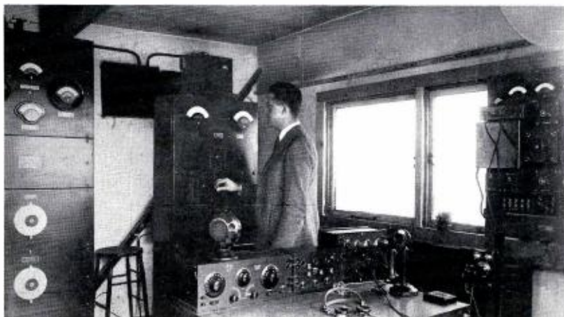
FIG. 5 (above). WOR's first transmitter installation on the roof of Bamberger's Department Store in Newark, February 1922. J. R. Poppele, engineer, at the controls.
