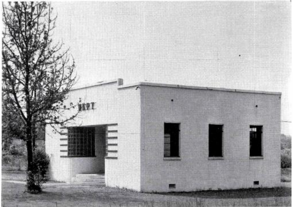
FIG. 7. The WKPT stuccoed tile transmitter building is located 2½ miles from Kingsport.
