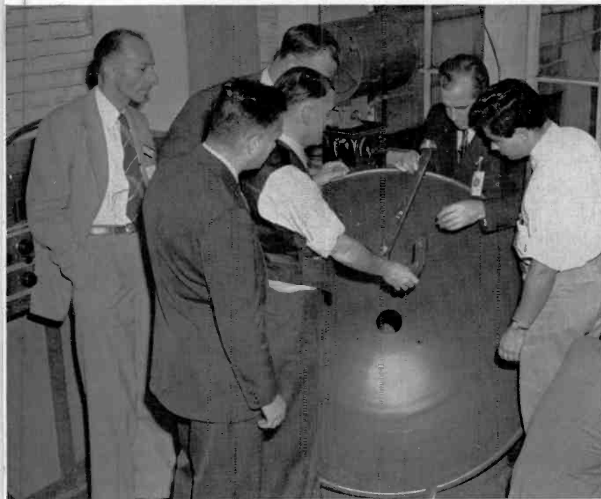
The hooked wave guide, parabolic reflector and control unit of an RCA Microwave relay transmitter are examined closely by the visiting engineers. From left to right they are: E. W. Lewis, WTVJ; H. E. Inslerman, Fort Monmouth, N. J.; C. Rosencrans, RCA Engineer,—behind him is F. V. Bremer, WAAT; R. Craig, WCAU; S. H. Barbour, RCA Engineer.
