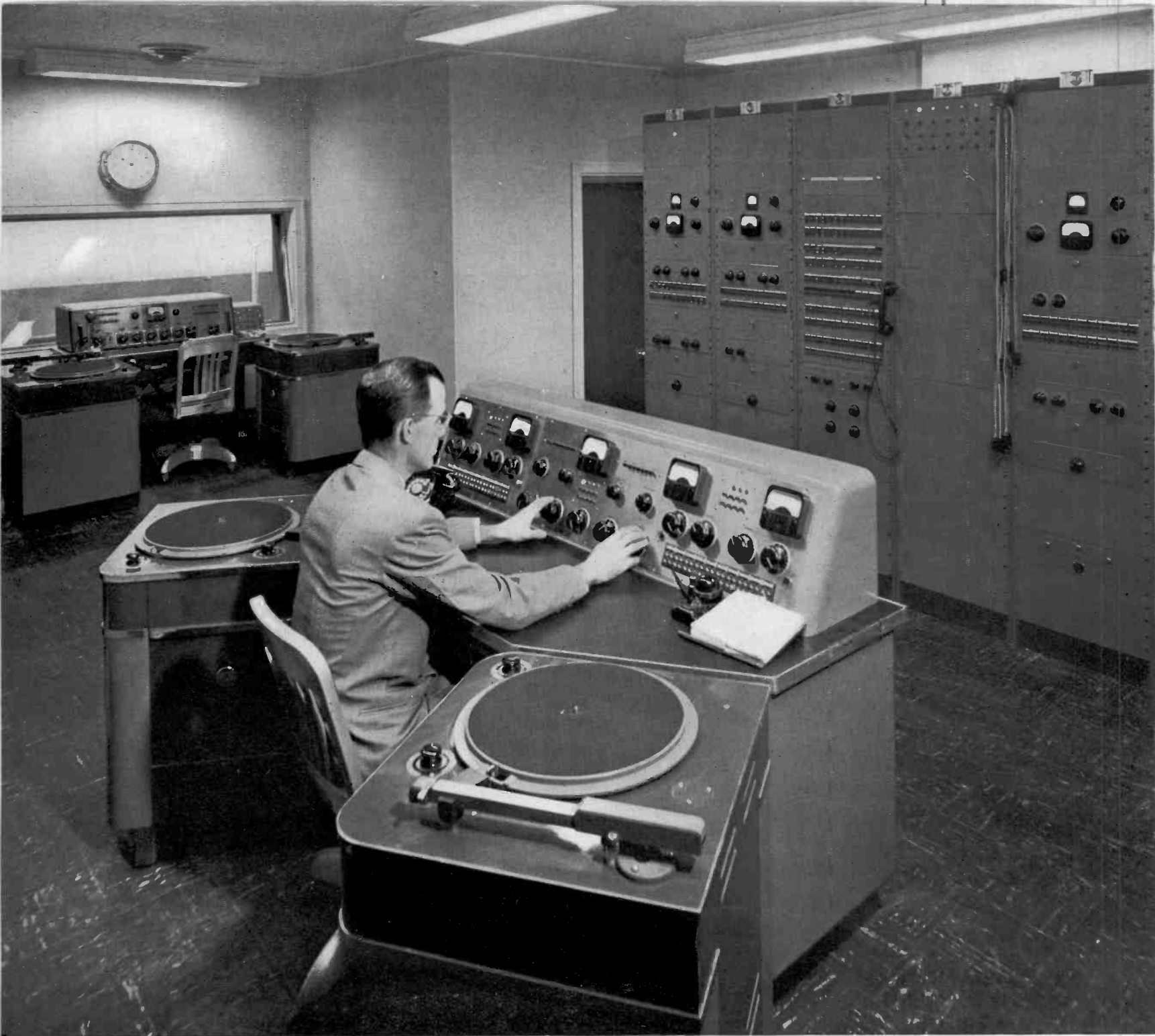
FIG. 1. Master control room of WBAL's new studio installation. R. S. Duncan, Chief Engineer of WBAL, at the control console.
