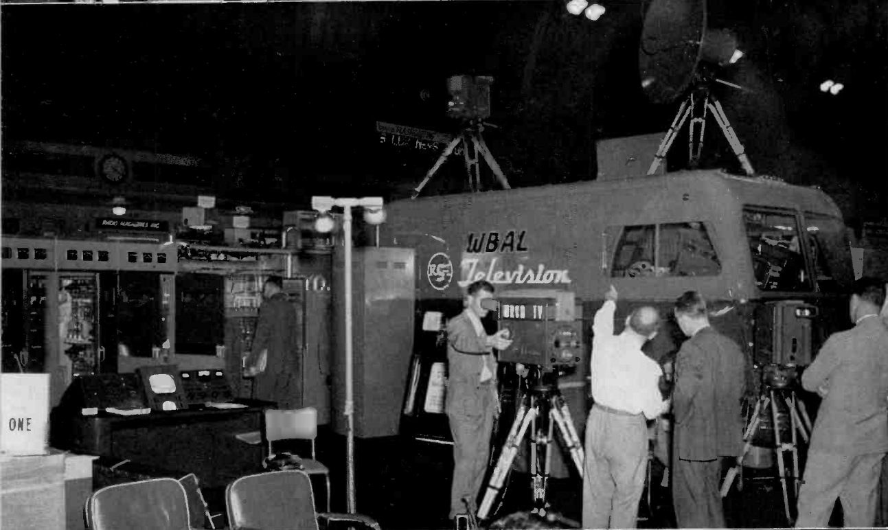
Biggest single item on the exhibit floor was this television mobile unit. Just out of the factory and completely equipped it was all ready for delivery to WBAL, Baltimore.
