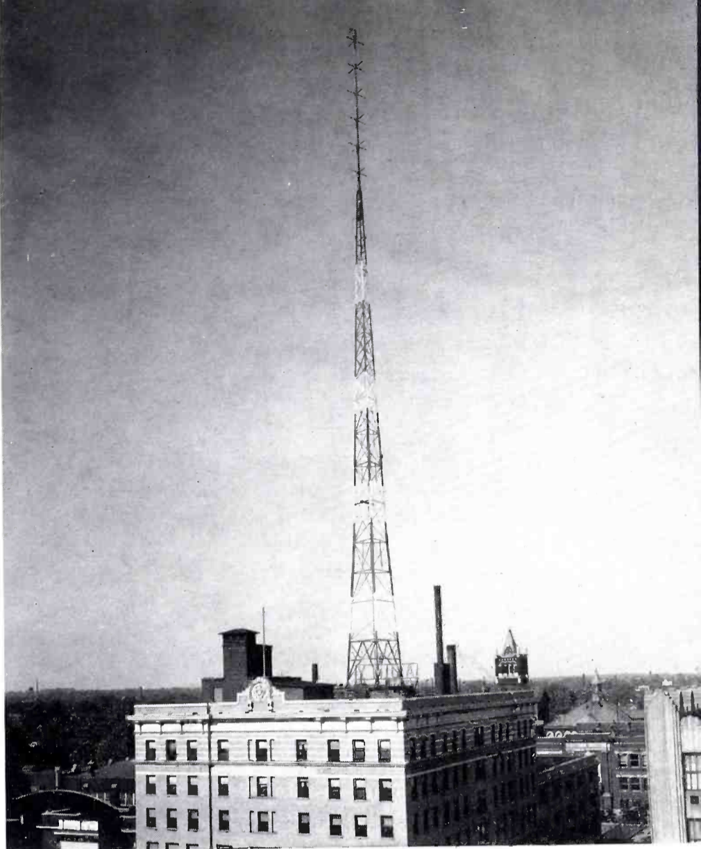
FIG. 8(d). ON A TOWER ERECTED ON A BUILDING. This is the antenna of WMLL, Evansville, Ind.
