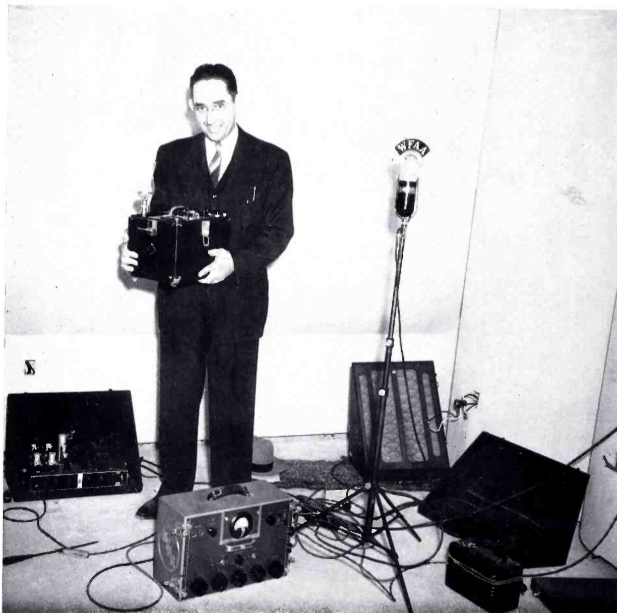
(Left) Dr. Boner with his reverberation measuring equipment set up in the studios at WFAA-KGKO, Dallas. Acoustical measurements were made at several stages of the construction. In this picture measurements are being made just before application of the floor covering.
