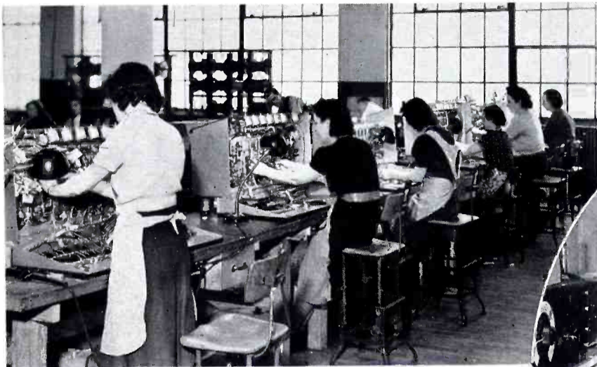
Assembling 76 B1 Consolettes.
