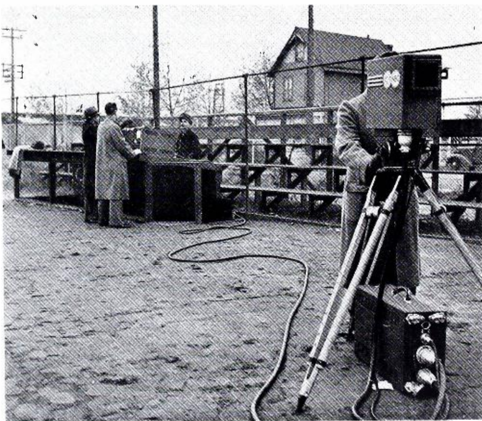
Camera set up in a typical operating position.
