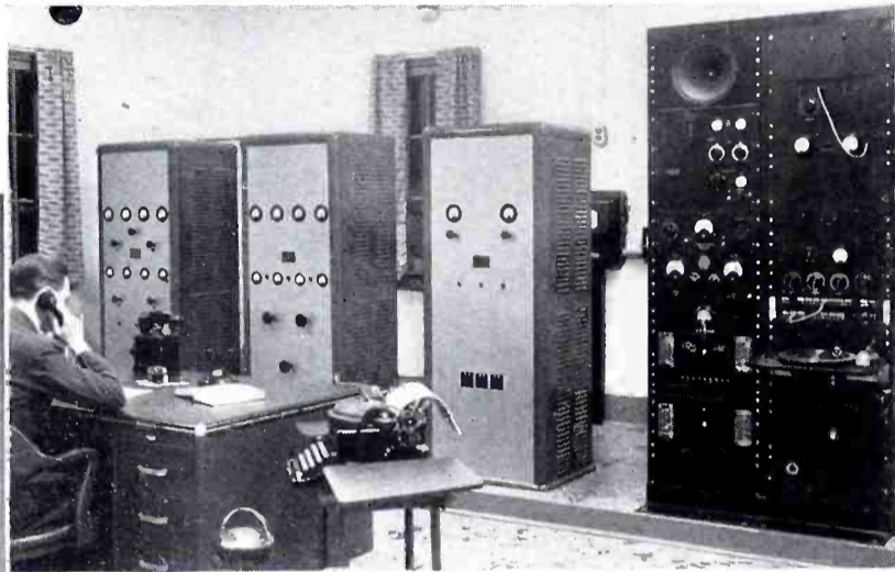
Above: CJKL—Kirkland Lake, Ontario, showing RCA 1-G Transmitter.
