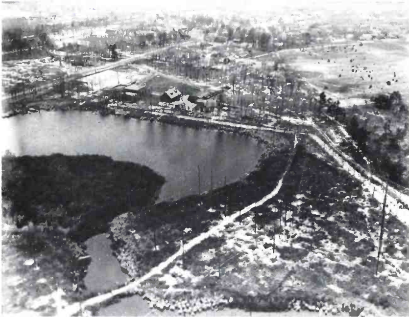
Aerial view of long wave and frequency measuring center.
