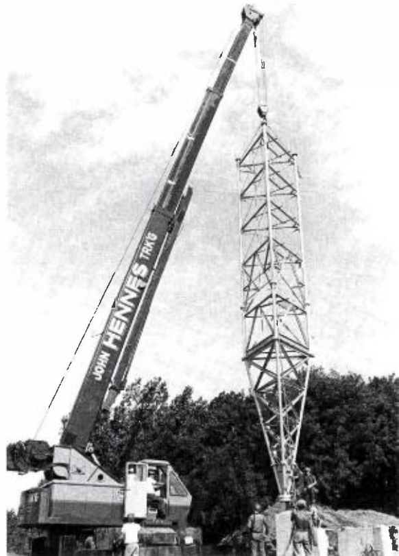
First section of tower is moved into position on the base.
