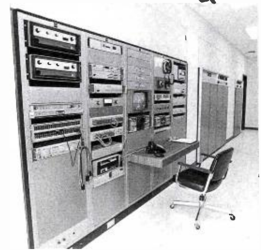
Monitor and control facilities for Ch. 18 and front line cabinets for TTU-55 transmitter are built-in for aesthetics and sound deadening.
