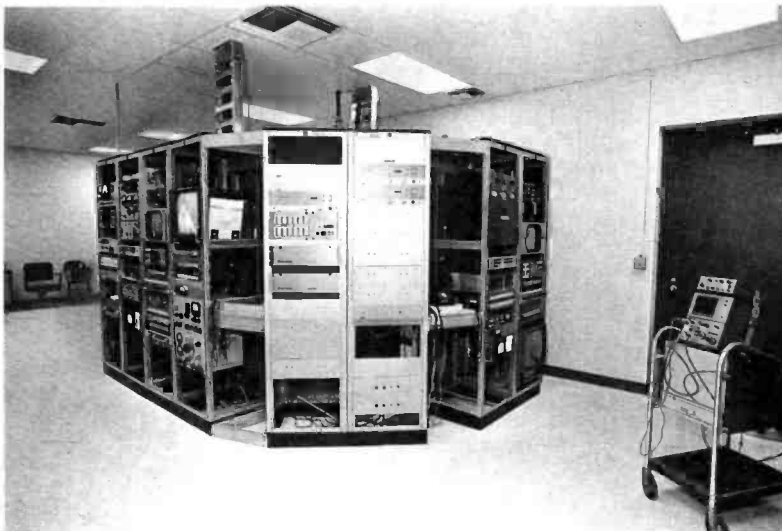
WMVS/WMVT share transmitting space, with their TT-35FH, 35 kW VHF transmitter and TTU-60D, 60 kW UHF transmitters also sharing monitoring and control facilities.
