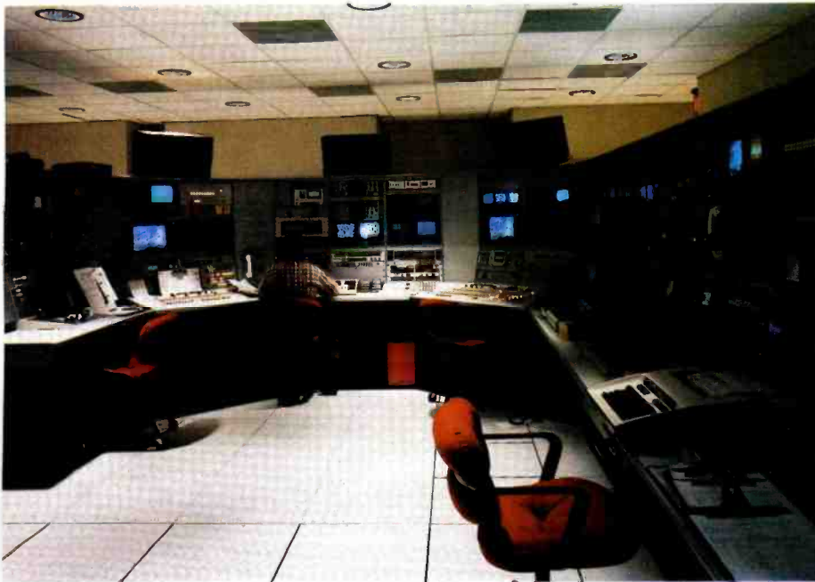
A new Transmitter Remote Control system and a computer-based control and monitoring system are a part of the Master Control Console.
