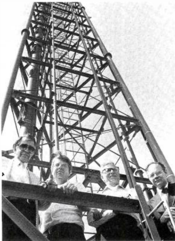
Standing on catwalk at the tower base are Bill Witt; Director of Engineering and Dennis Brechin, Transmitter Supervisor for WVTV; Gino Monaco, Transmitter Supervisor, and Harold Wagner, Chief Engineer for WMVS/WMVT.
