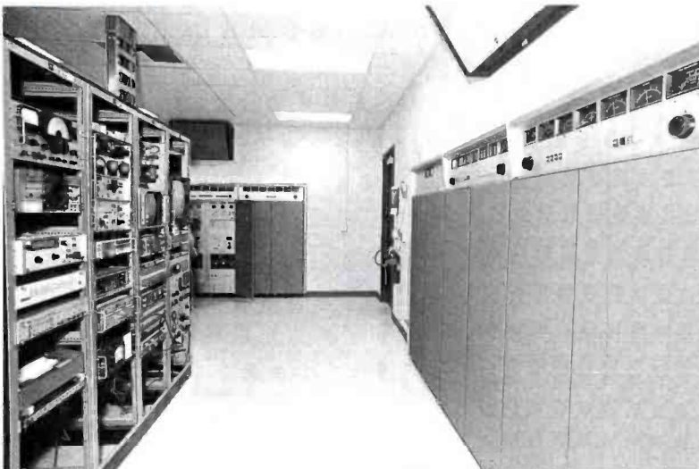
WMVS/WMVT share transmitting space, with their TT-35FH, 35 kW VHF transmitter and TTU-60D, 60 kW UHF transmitters also sharing monitoring and control facilities.
