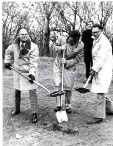
Breaking ground for the new tower on March 31, 1980 are (left to right) Harold Wagner, Chief Engineer for WMVS/WMTV; Joseph Loughlin (then General Manager of WVTV), and Bill Witt, Director of Engineering for WVTV.
