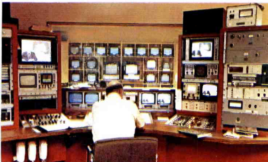
A window in front of the Master Control operator looks in on Production Control with its banks of video source monitors.
