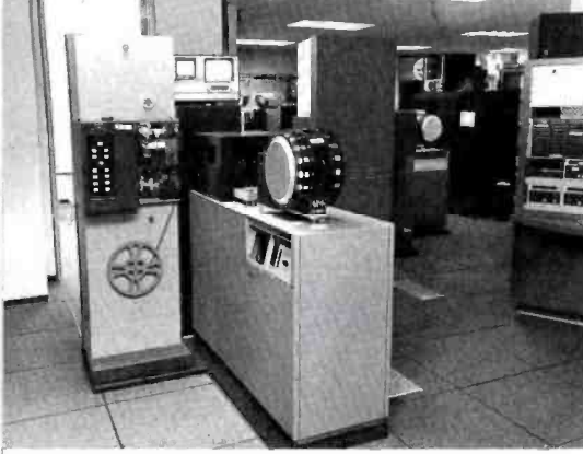
Film islands and other equipment are on computer flooring, with access from all sides.
