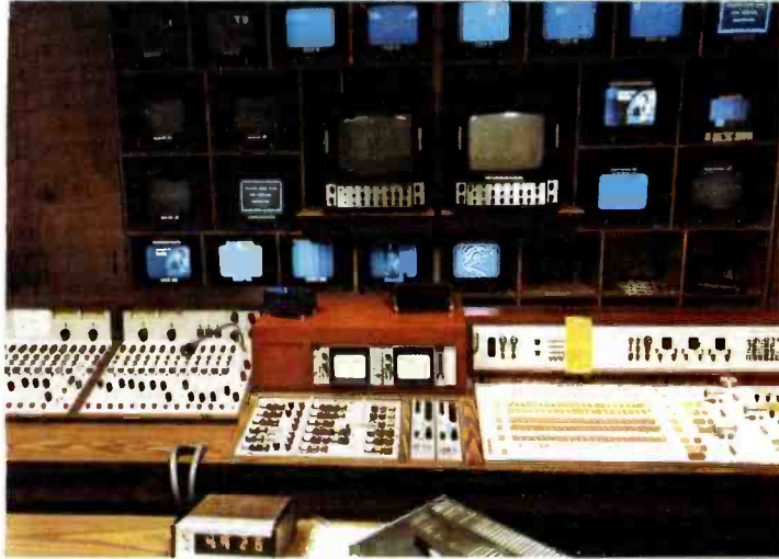
Production Control is on two levels, with audio and video switching and remote machine controls at the lower level.
