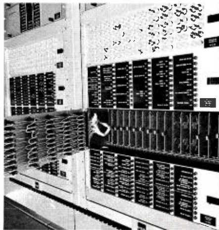
Status interface panel in open position. At bottom is a fuse panel through which all metering inputs are routed before passing into the system.
