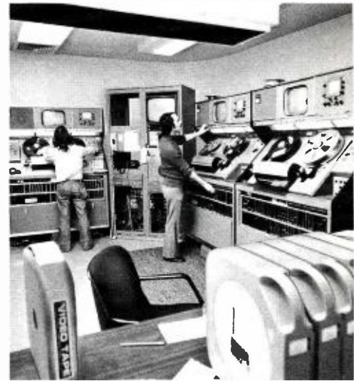
Three of seven TR-70C's are reserved for major editing work. Global has parlayed a built-in VTR advantage into an economical, home-grown editing technique allowing consistent edits within a quarter second of that obtained with expensive edit controllers.
