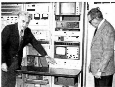
Jerry Klabunde, Technical Director, WBEN-FM/AM is shown in the AM studio with the unusual remote control arrangement which he devised. Just above the console is a U-shaped unit housing all remote control equipment. A winch, controlled by a switch on the console, raises and lowers the unit to a convenient height.
