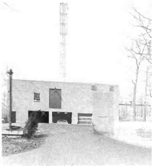
The new TT-35FH Transmitter is located on this addition made to the Hellam building.
