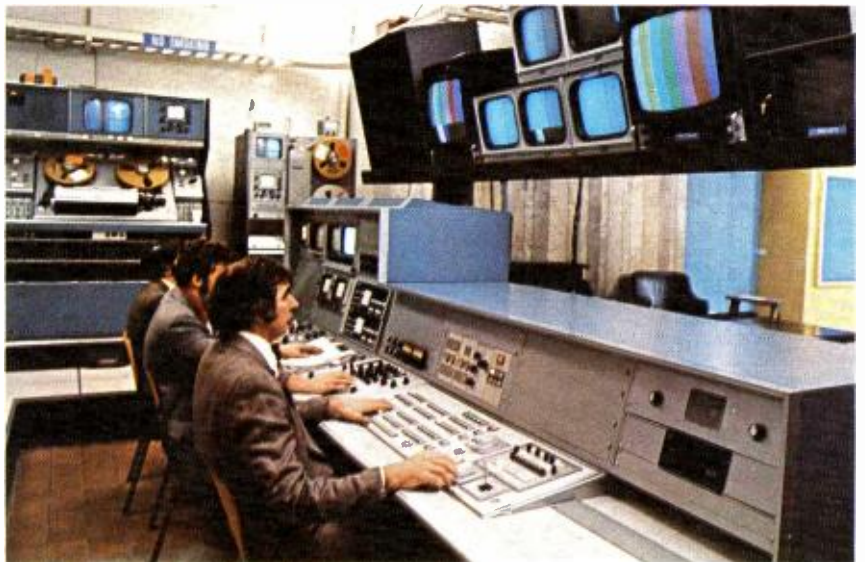
The Control Room is adjacent to the studio. All of the racks and equipment are mounted on a computer floor, making for a neat, efficient installation. Production is normally handled by a three-man control room crew: A Director who does his own switching. One man operates the TR-70 and TR-60 VTR's (both are used in original recording) from the remote panel of the Time Code Editing console—and also rides audio levels. The third crew member shades the TK-44B's via joy stick remote controls.
