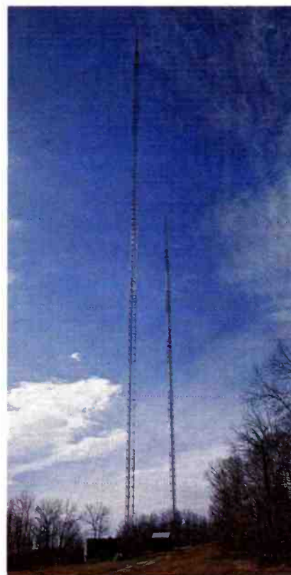
The new 747-foot tower topped with the 76-foot Traveling Wave Antenna is seen next to the old Superturnstile Antenna, which stands 502-feet above the ground.
