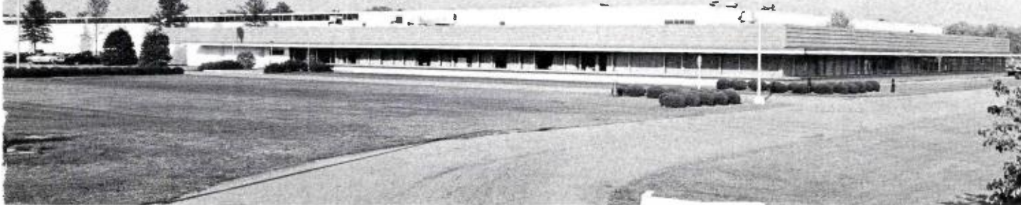
Modern Parts and Accessories distribution center at Deptford, N. J. Giant 26-acre building is located within easy reach of rail, truck and air transportation facilities. Philadelphia's International Airport is only 15-minutes away.
