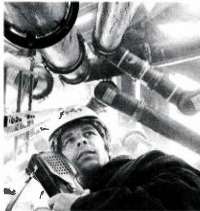
TWO WAY RADIOS provided voice contact between crews aloft and ground during construction. Permanent intercom system was installed later.
