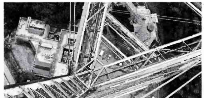
TOP TO BOTTOM. Photo taken from the top level looking down the tower shows the roof of the transmitter building at the base (left) and Sutro Mansion (right center).
