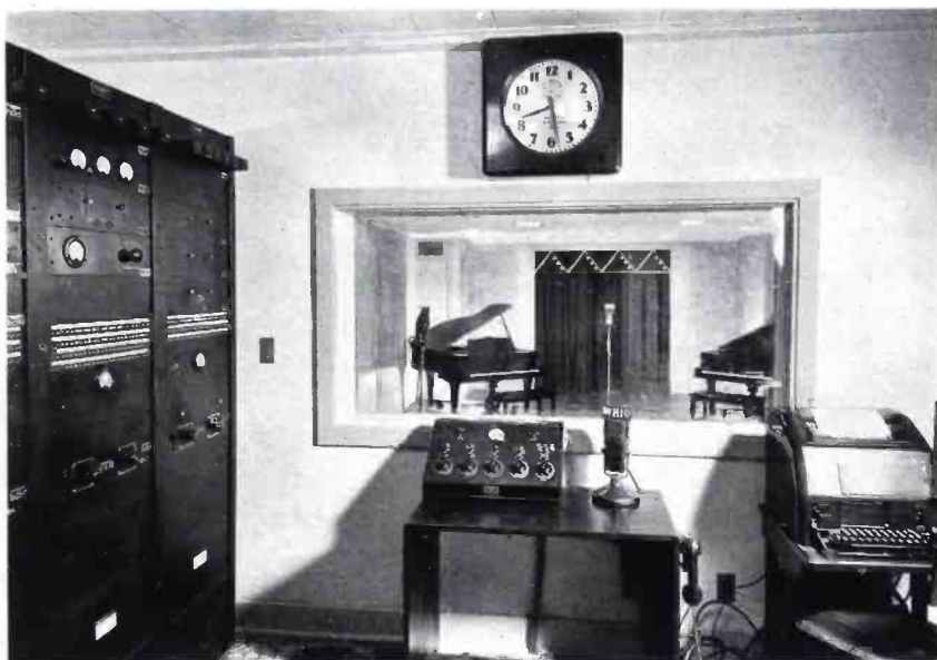
VIEW FROM MAIN CONTROL ROOM, THROUGH SOUND-PROOF WINDOW, INTO THE SALON STUDIO. RCA SPEECH INPUT EQUIPMENT IS SHOWN AT THE LEFT AND IN THE CENTER FOREGROUND, AND THE TELETYPE EQUIPMENT IS LOCATED AT THE RIGHT
