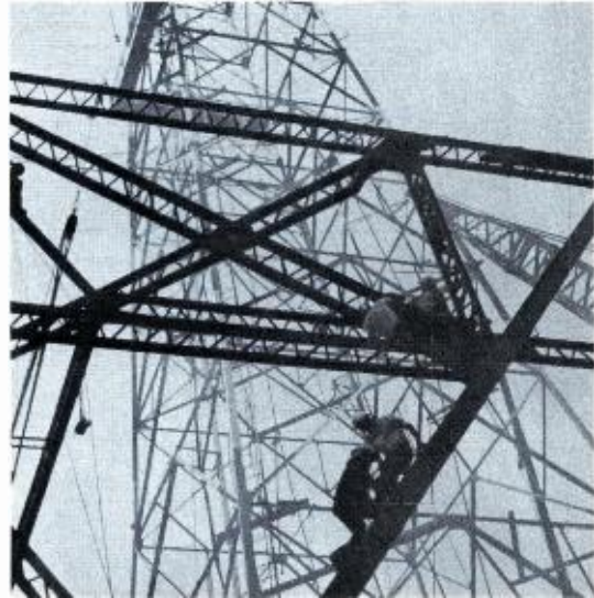
In the background is the new, 650-ft., tower being built around the existing structure.
