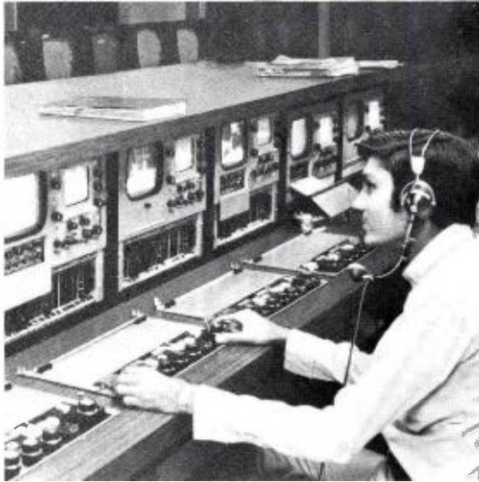
TK-44A Camera Control Units (CCU's) in the centralized video control center.
