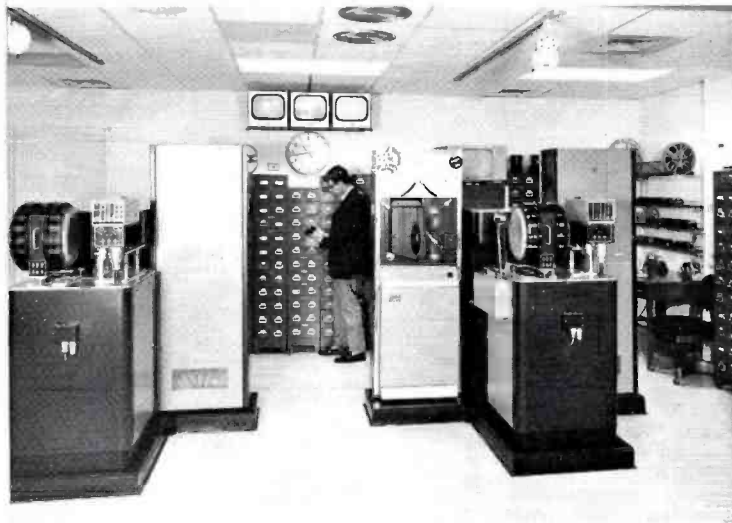
FILM AREA includes two film islands, storage and film editing facilities. Latest-design equipments for color and monochrome include a TK-27 4-vidicon color film chain and two TK-22 monochrome film chains.
