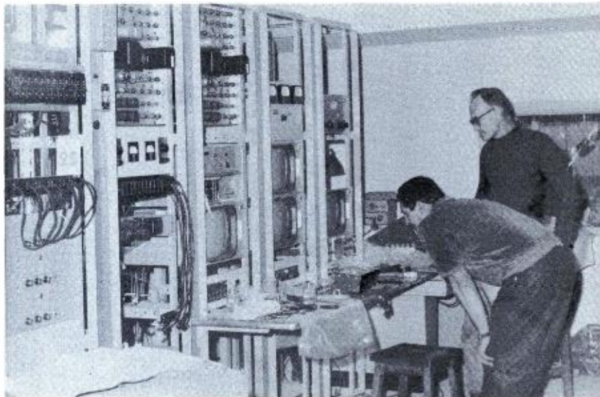
FIG. 7 Installation of terminal and control equipment.
