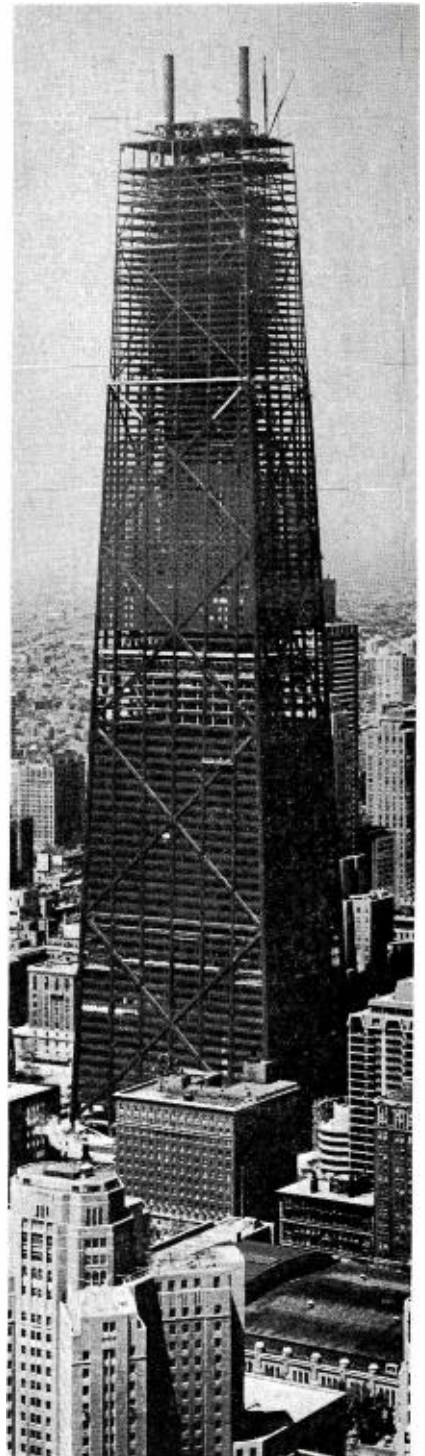
TV antennas will be mounted on twin tubes rising from 'Big John's' roof. Drawing at left shows configuration of antennas.
