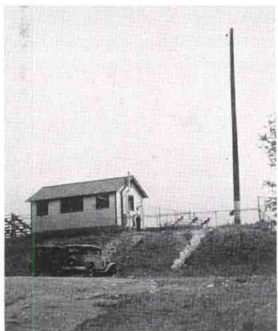
THIS LITTLE SHACK IN WOODSIDE PARK, PHILADELPHIA, SERVED IN 1930 AS THE HOME FOR BOTH THE TRANSMITTER AND STUDIO OF WPEN, WHERE THE S. S. "ALL IN FUN" HAD ITS MODEST BEGINNING
