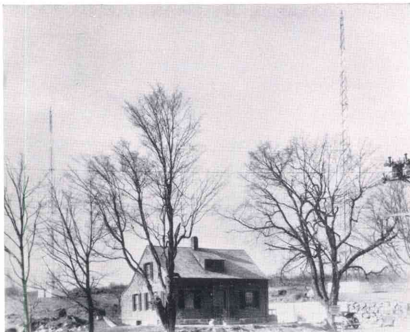
THE TRANSMITTER HOUSE OF W1XBS, AT PROSPECT, CONN., SHOWING THE TOWERS IN THE BACKGROUND
