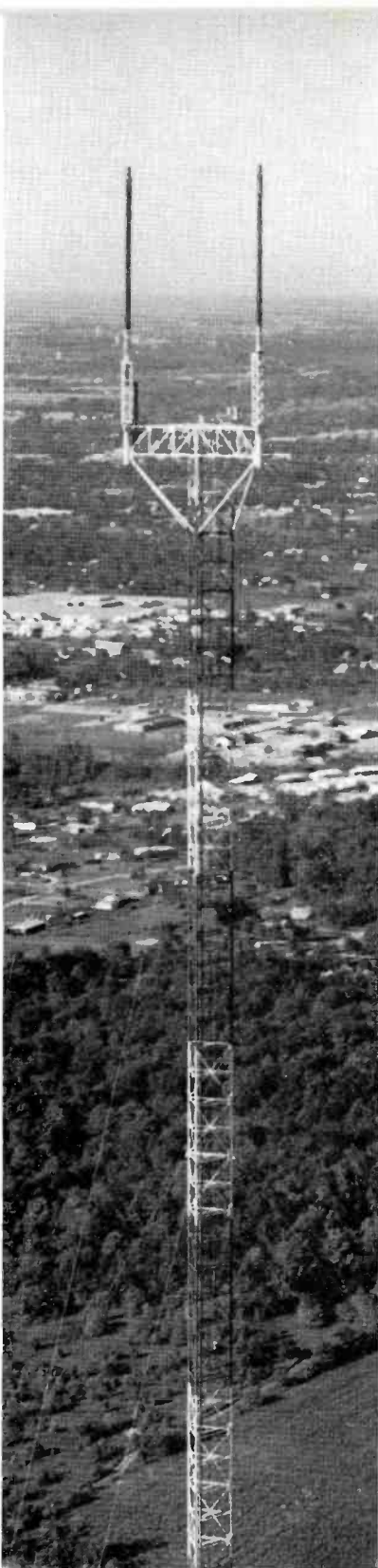
FIG. 3. "30J" Pylons of stations WKBD-TV and WTVS, Detroit.
