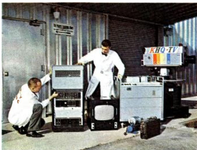
Scene at KHQ-TV loading dock as TK-42 and TR-5 are loaded into panel truck that serves as mobile unit.
