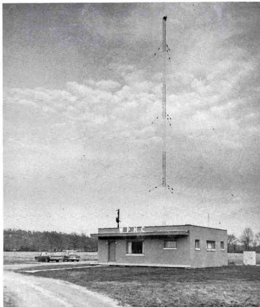
FIG. 2. WPHC's brick-veneered concrete-block building houses all facilities of the station. The antenna tower is just four feet from the rear of the building. Utility power enters the building underground.
