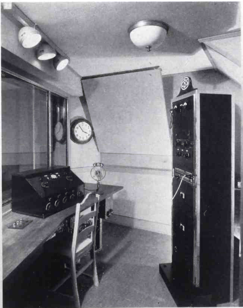
INTERIOR OF COLUMBIA'S NEW CONTROL ROOM AT DETROIT ORCHESTRA HALL— RCA VICTOR EQUIPPED
