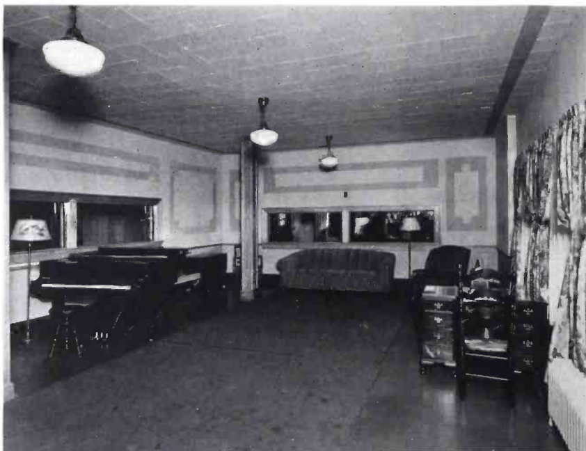
STUDIO A (20 BY 36 FEET), LOOKING TOWARD CONTROL ROOM. RADIO STATION WTAR, NORFOLK, VA.
