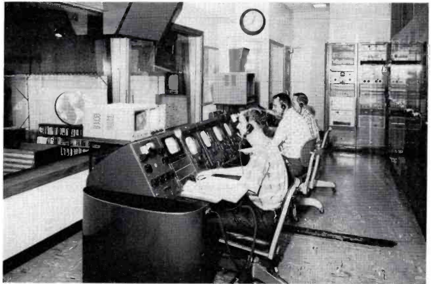
▲ FIG. 6. Master Control room of KTTS-TV.
