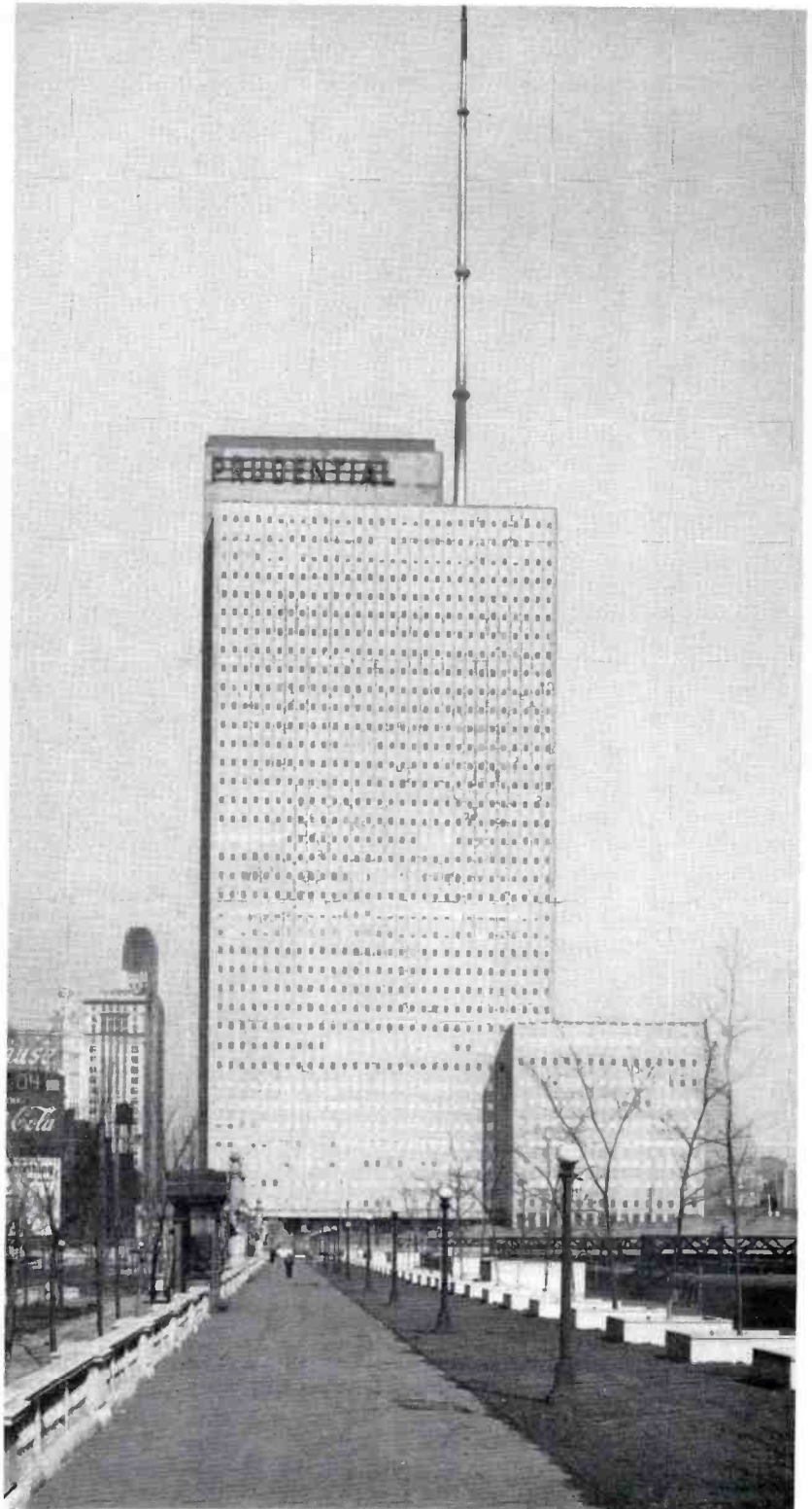
FIG. 22. Prudential building in downtown Chicago houses WGN television transmitter. It also supports attractive tubular steel tower with superturnstile antenna.
