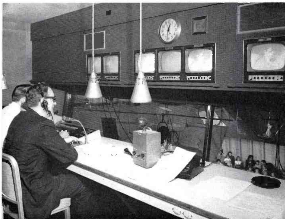
FIG. 13. Control room, 15 ft. above studio floor, gives good visual coverage of studio.
