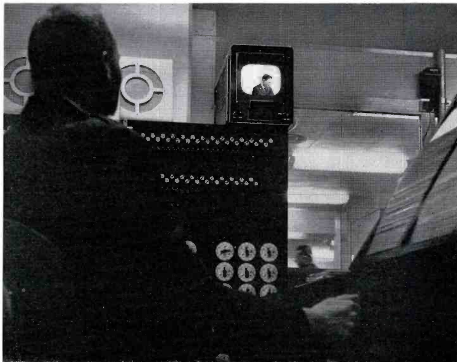
FIG. 20. SAC operations control room personnel identify visitors outside area via this TV control monitor. When positive identification is made, the operator allows the visitor to enter by pushing a button, automatically opening the door to the area.
