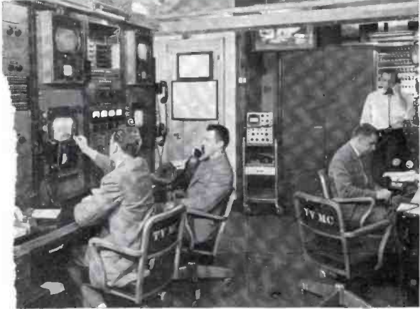
NERVE CENTER of ABC-TV operations—the master control room—is largely RCA equipped.
