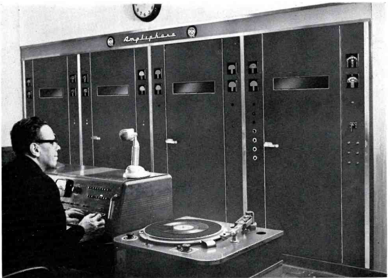
FIG. 10. Alfred Jorgenson, WINS Transmitter Engineer, is shown at the 76B Console in the transmitter building. One of the 70C Turntables is on his right. The input and monitoring equipment is to the rear within arm's reach. This console and turntable can be used to originate programs at the transmitter site.
