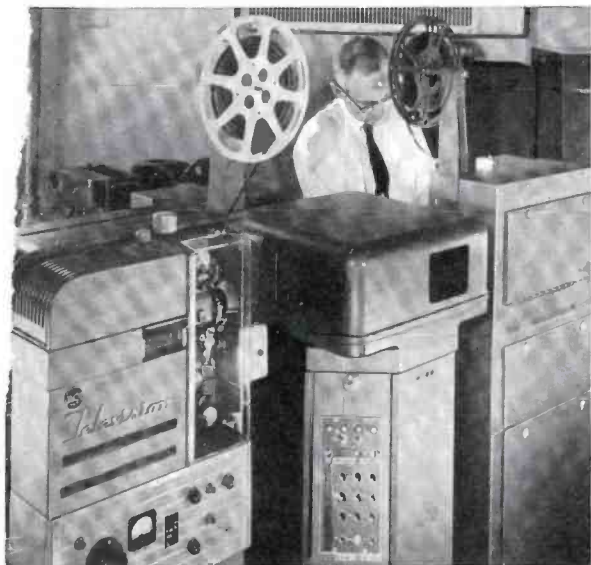
PROTECTION SYSTEM. RCA TP-6 16 mm professional projectors are used to double-up with 35 mm network projectors to insure on-air continuity in event of mishap. TP-6's are used throughout ABC local film rooms.
