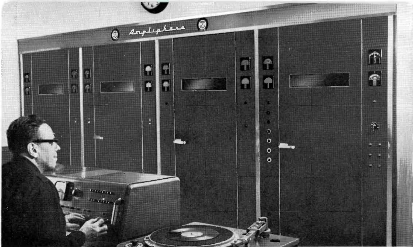
RCA Type BTA-50G transmitter at the WINS transmitter building in Lyndhurst, New Jersey, showing Al Jorgenson at Console.
