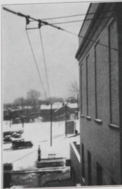
TRANSMISSION LINE BETWEEN TRANSMITTER AND ANTENNA, AT WPET, NEWLY INSTALLED RCA VICTOR POLICE RADIO STATION AT LEXINGTON, KY.
