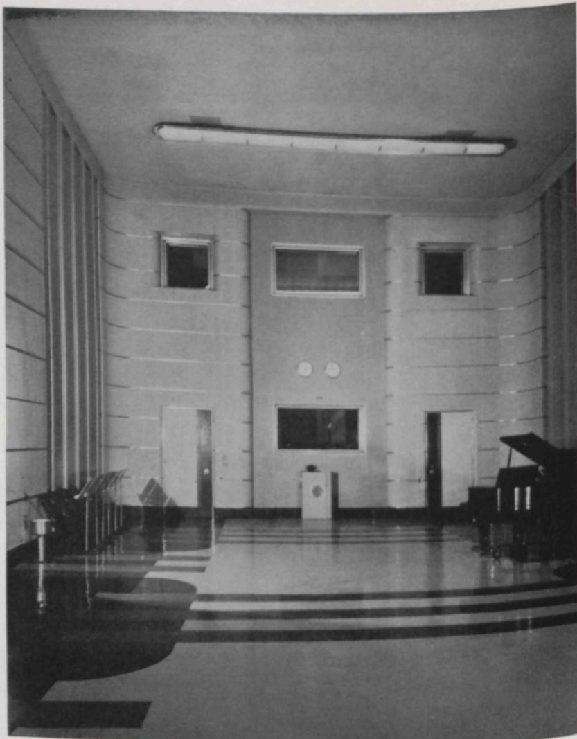
STUDIO A, LOOKING TOWARD THE "LIVE END." THE THREE SOUND PROOF WINDOWS AT THE TOP PERMIT VISITORS TO OBSERVE THE PERFORMERS AND THE CENTRAL WINDOW BELOW SEPARATES THE LOCAL CONTROL OPERATOR FROM THE STUDIO. THE MASSIVE SOUND PROOF DOORS AT THE LEFT AND THE RIGHT EACH WEIGH 600 POUNDS. THE LOUDSPEAKER BELOW THE CONTROL OPERATOR'S WINDOW, AND A SPECIAL MICROPHONE FOR THE PURPOSE, PERMIT TWO WAY CONVERSATIONS WHEN DESIRED BETWEEN PERFORMERS IN THE STUDIO AND THE OPERATOR IN THE STUDIO CONTROL ROOM.
