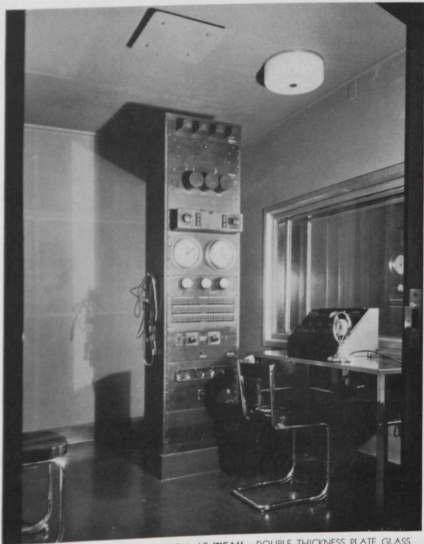
A TYPICAL STUDIO CONTROL ROOM AT WCAU. DOUBLE THICKNESS PLATE GLASS WINDOWS, SEPARATED BY SUITABLE AIR SPACE, COMPLETE THE SOUND PROOFING USED IN THE CONSTRUCTION OF THIS CHAMBER. THE CONTROL DESK AND THE PANEL-MOUNTED EQUIPMENT PROVIDE THE MOST UP TO DATE MEANS FOR CONTROLLING AND MONITORING AND FOR PASSING THE PROGRAM ON TO THE MASTER CONTROL ROOM AND THENCE TO THE REMOTELY LOCATED TRANSMITTER.
