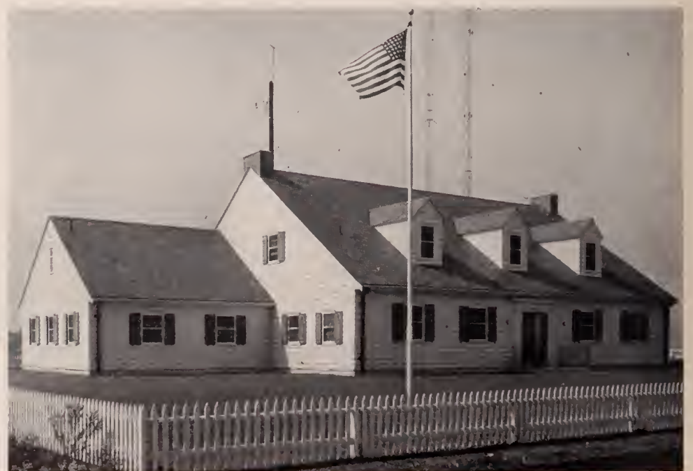
WBZ's Cape Cod "Dwelling" Transmitter House at Hull, Mass.
