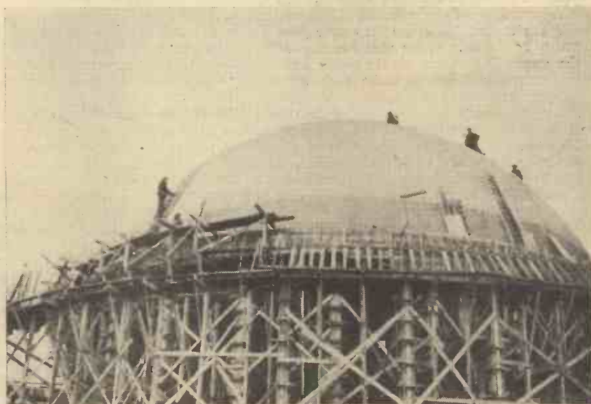
The Palace of Science in course of construction
