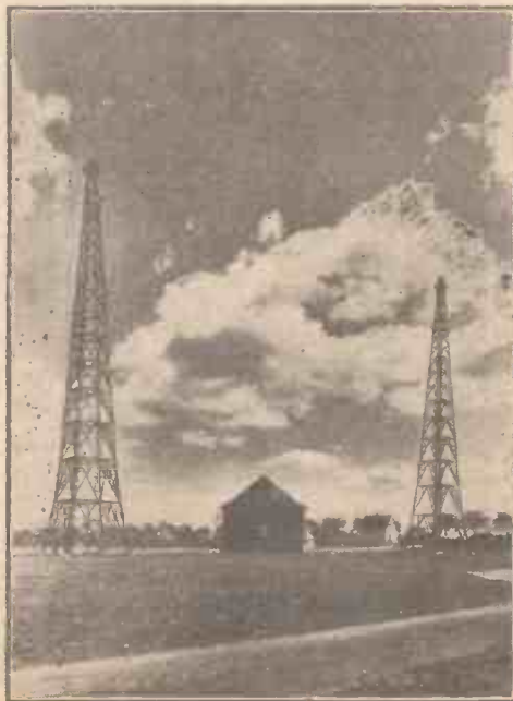
The Aerial masts, Flensburg Station.
