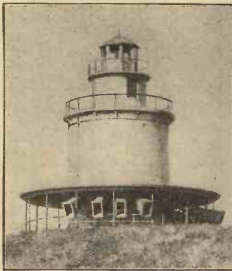
The odd structure above serves, not only as a lighthouse, but also as a community radio loud speaker. It is located at Dartmouth, Mass., where the Round Hills Radio Corporation maintains station WMAF. Around this battery of huge speakers the whole population of the town may gather on pleasant evenings to hear programmes reproduced with a volume that fills all outdoors.
