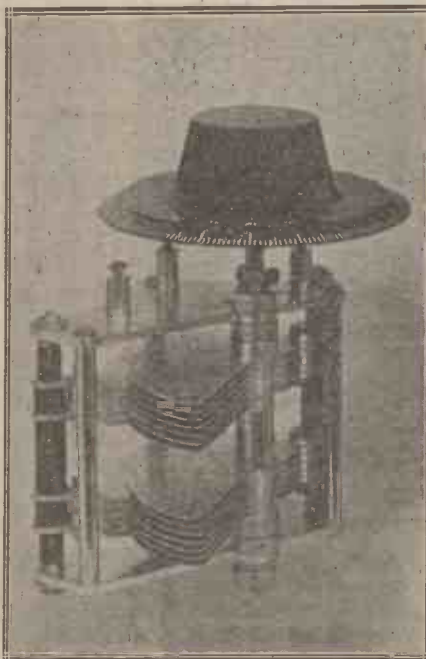
The use of double condensers for the simultaneous tuning of two circuits involves many problems concerning the shape of the plates.
