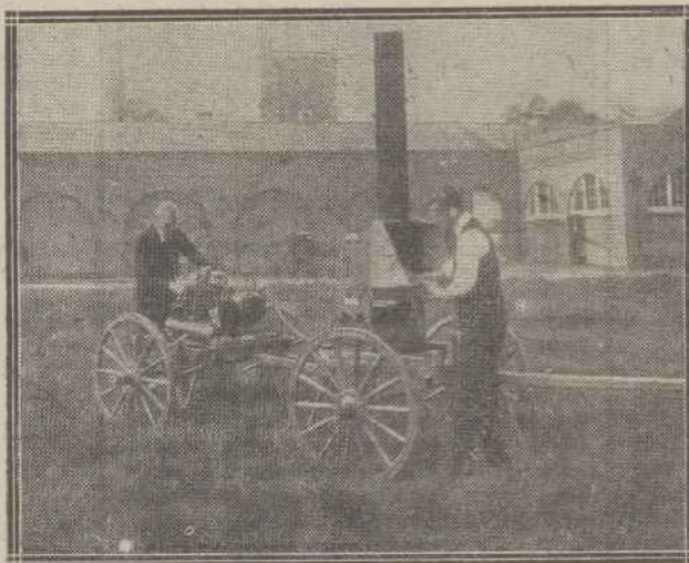
Rapidly transported wireless sets play a vital part in modern warfare. The photo shows one of these equipments undergoing its final tests. A petrol motor supplies the power.
