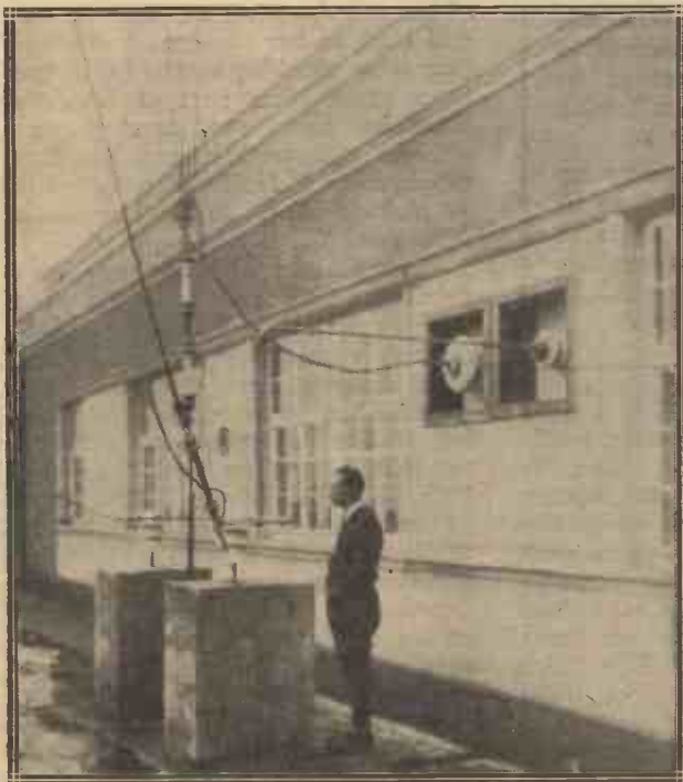
The leading-in point of the aerial and counterpoise at the new high-power Rosenhugel broadcasting station, near Vienna.
