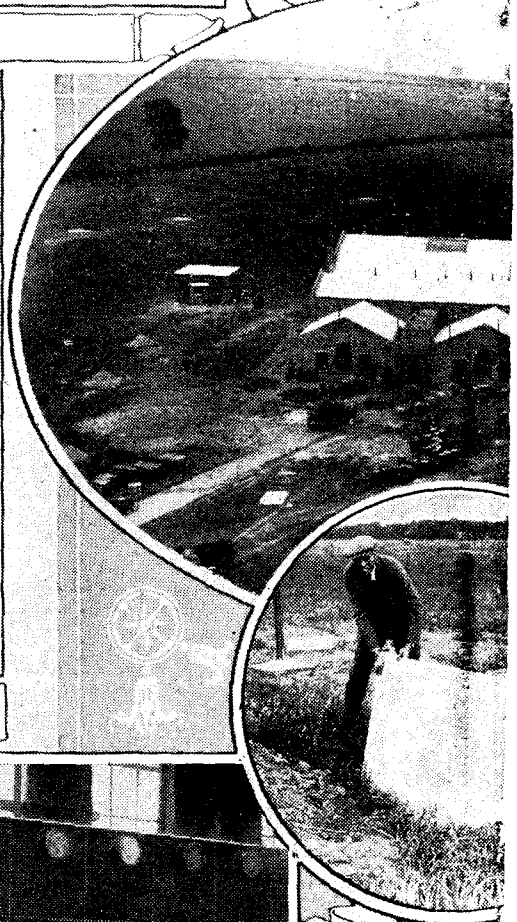
Lowering one of Earth Plates
