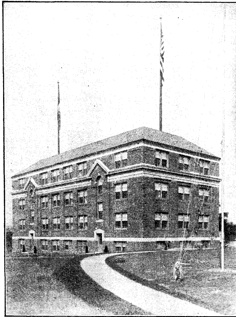
The Radio Corporation technical building at Van Cortlandt Park, New York. The masts support a single wire aerial.
