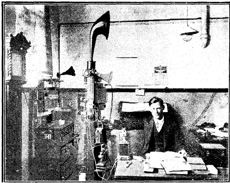
The control room at the Johannesburg broadcasting station.
