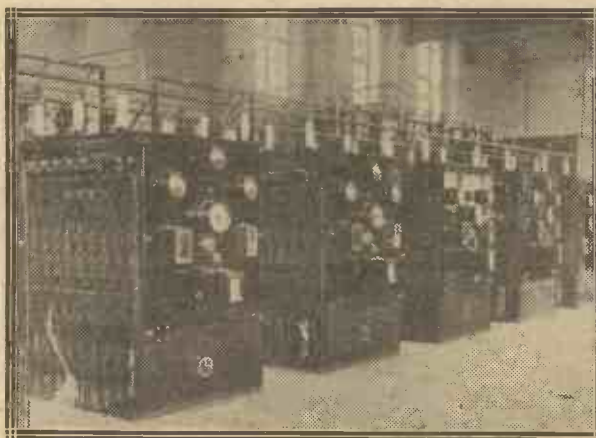
An interesting article appears elsewhere in this issue dealing with the Empire's Wireless system. This view shows the main valve panels at Rugby.
