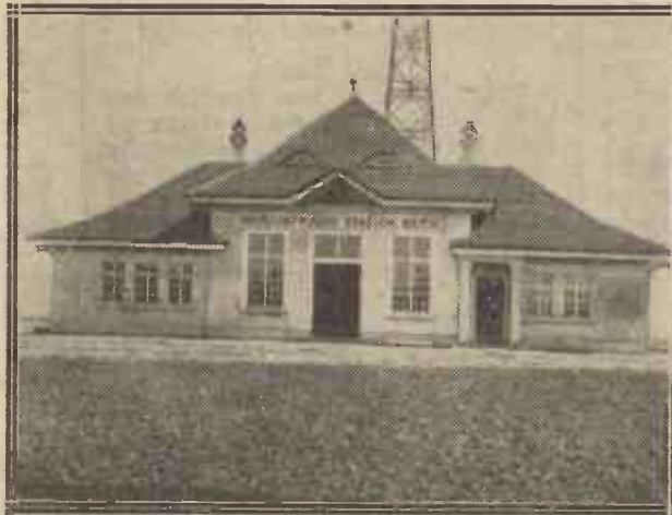
The Berne broadcasting station is one of the very few which possesses a real station building of its own.
