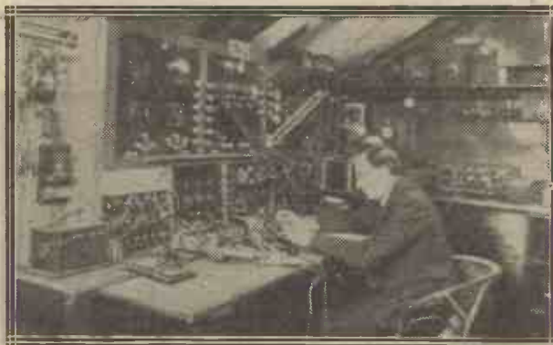
Mr. G. Pailin (6ZP) is experimenting on the control of electrical switchgear by radio. The above photographs show his apparatus and the aerial system in use.
