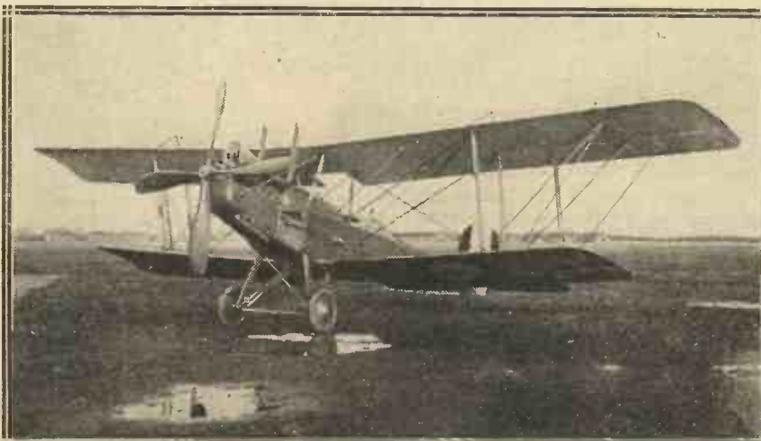
The R.E.S., a standard type of British Artillery Observation aeroplane used during the period 1917-1918. The engine was the 150 h.p. Government designed Royal Aircraft Factory, Raf 2a, and was air cooled.
