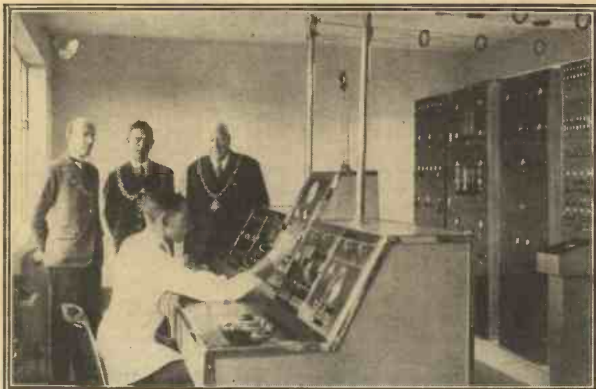
The mayors of Ramsgate and Margate and the senior councillor of Broadstairs recently jointly declared open the first building erected for the sole purpose of housing the complete equipment for the reception and redistribution of broadcast programmes under the popular relay system. The relay in question is that in operation in Thanet and the building is conveniently placed for serving the three adjacent towns.
